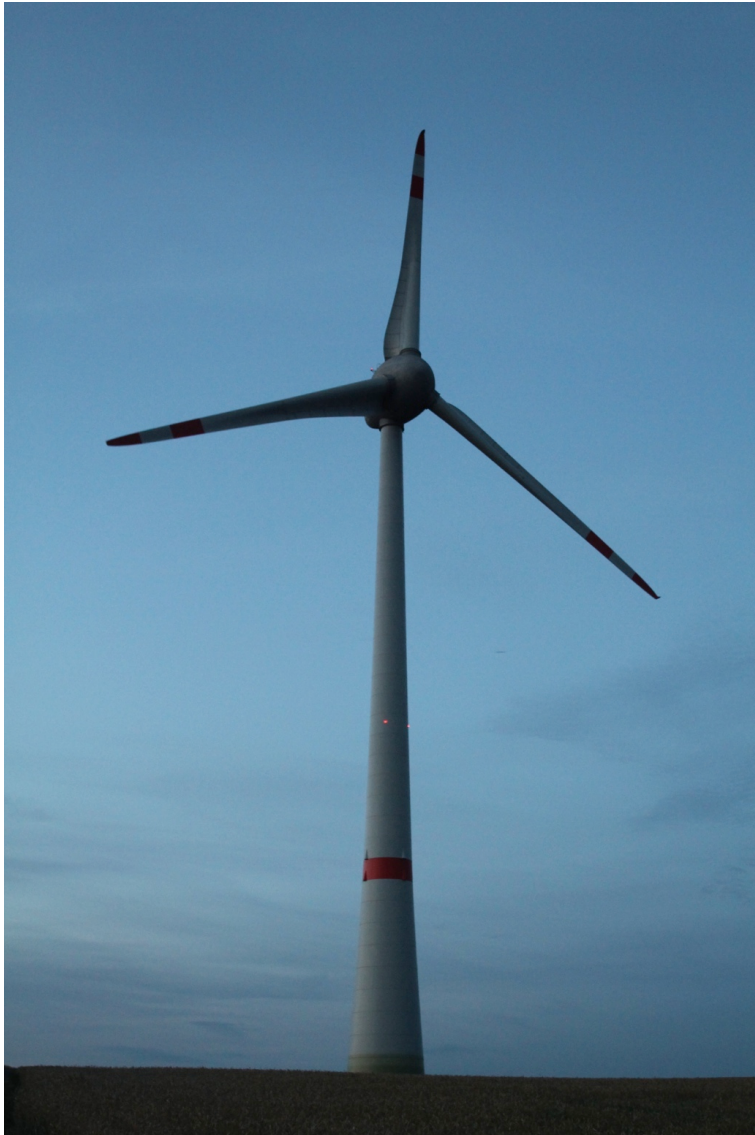
Enercon E-126 – 7.6 MW – worlds largest wind turbine Tower 135m / Total 198.5m / Blades 56m / Hybrid
